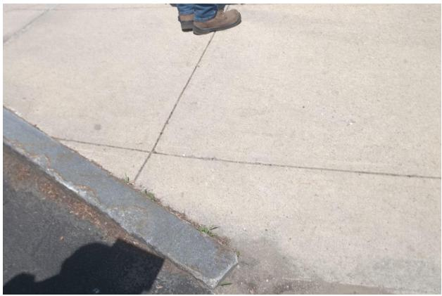
The ADA Team determined that the curb cut to the sidewalk that leads to the accessible entrance to the Library from the parking lot needs repair or patching. We recommend that the curb cut be repaired to improve the accessibility to the Groton Public Library's accessible entrance. An example of such a tactile warning is included with this report.
